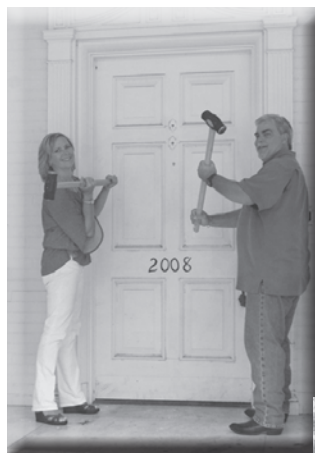
Tami and Robby Burdge, Capital Campaign Co-Chairs take the first hit of demolition.
