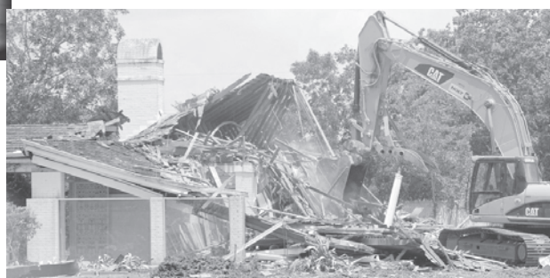
Right, construction crew tears down the pool house.
