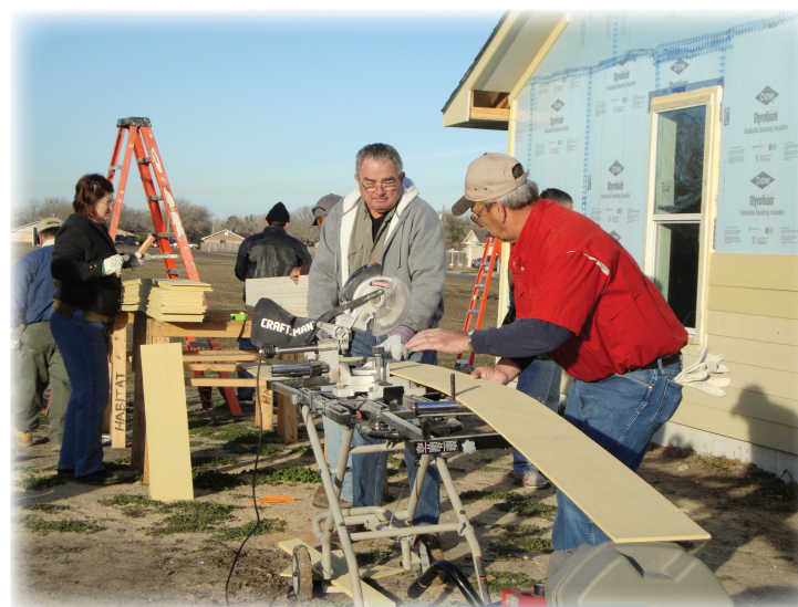
(above) KC Council #9088 members, George Wenzel and Lee Pribyl, prepare siding to be nailed to the outside wall of the 75th Habitat for Humanity Home built in Victoria.
