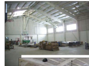
Below: Work being done on new gym
