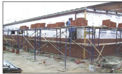
Above: Bricks being laid on new Fellowship Center
