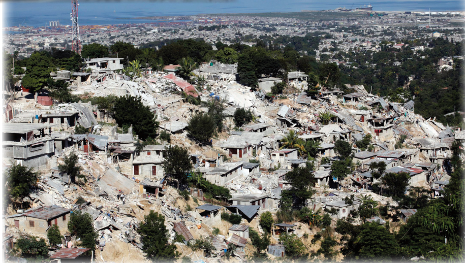
(above) Destroyed houses are seen in a view of the Canape-Vert area Jan. 13 after a massive earthquake struck Port-au-Prince, Haiti. The Red Cross said one-third of Haiti’s population will require aid following the devastating quake. (CNS photo/Eduardo Munoz, Reuters) (inset) Children walk among tents in a makeshift camp at a golf course in Port-au-Prince, Haiti, Jan. 24. The Haitian government said as many as 1.5 million people were left homeless by the catastrophic Jan. 12 earthquake. (CNS photo/Marco Dormino, United Nations via Reuters)
